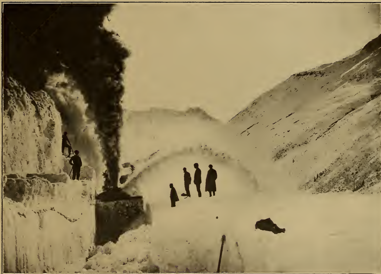
CLEARING TRACKS ON W. P. & Y. R. R.
